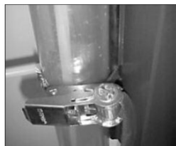
Fasten ratchet strap to well
